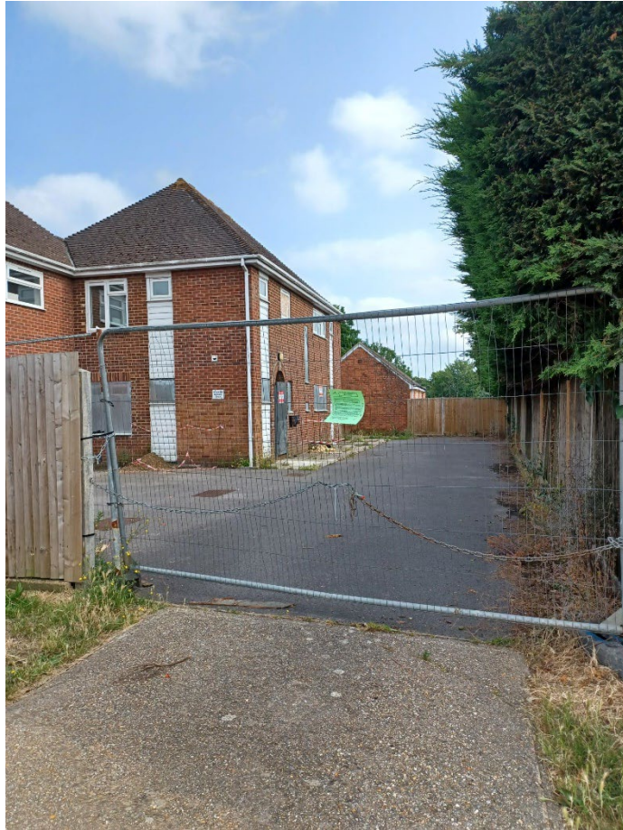
Access to the site
